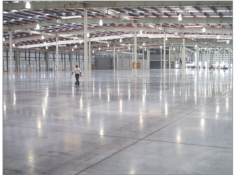
Distribution Facility, Guadalajara, Mexico
